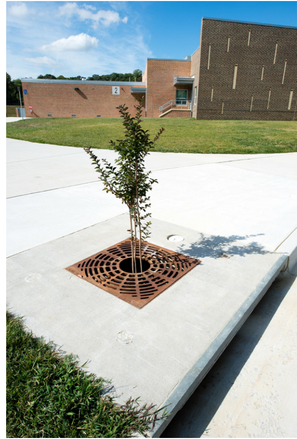
Filterras® storm water bio-filtration systems are installed to filter pollutants from stormwater at renovated schools' parking areas.
