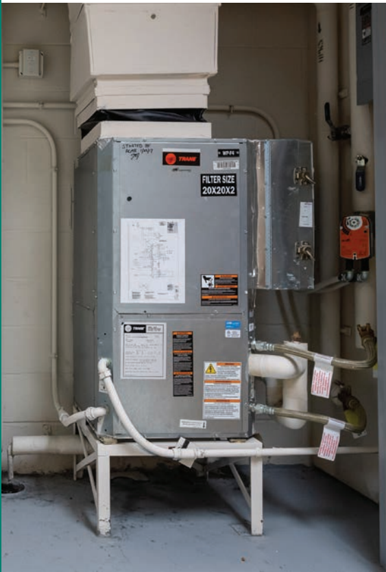
Ground Source Heat Pumps heat and cool using the constant temperature of the earth extracted from wells hundreds of feet deep for the source of heat transfer.
